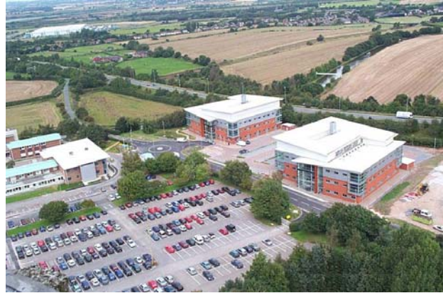
Picture Above: View of Keckwick Lane mini-roundabout access to existing car park, new building entrance and new building car park.
